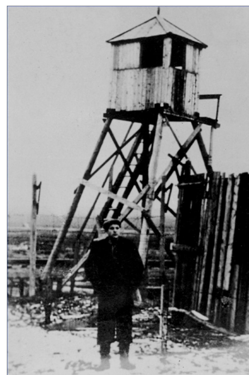
Wachturm in Workuta
